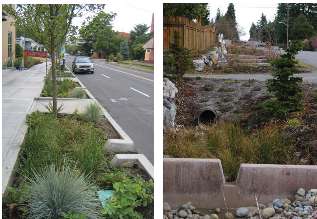
Image 2. 3. Evolving filtration stormwater BMPs along roadsides Image source: Stuart Echols
